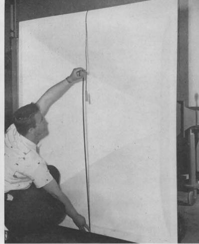
LARGE HORN AND DRIVER for the Acoustic Facility is checked out by Ed Buksa, left, and John Colburn prior to installation for a test. Microphone is positioned to check the sound intensity level pro-
